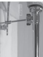
Replace existing ball rod gasket or choose one of the included gaskets that best fits the port. Missing or damaged gasket can cause leak. Install new ball rod and tighten nut.
