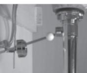
Disconnect linkage, loosen the ball rod nut and discard the existing ball rod. Save the existing nut and ball rod gasket.
